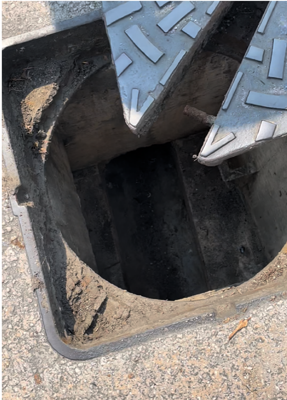
Photo showing the internal of existing manhole to be connected
